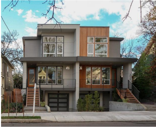
Figure 19.35.020.B2. Examples of elevated ground floors to allow partially below-grade garages that do not count against habitable space requirements. Image Credits: Zillow.
